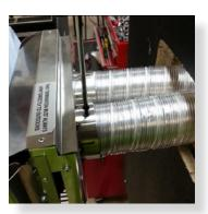
Feed air intake flue into connection, ensure inserted 50mm. Fit retaining screw from below.
