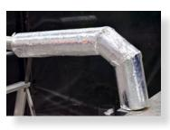
Bends were practical should be insulated, by cutting the insulation into segments and taping together.
