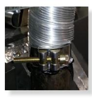
Slide flue onto connection spigot fully.
