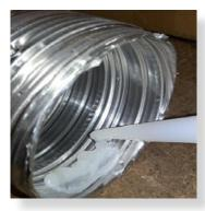
Apply an 8mm silicon bead fully around the inside of the flue end (heater connection end)
