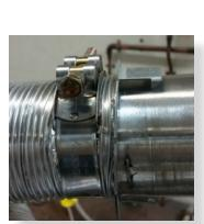
Fit flue clamp over flue (loosely).
