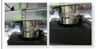
Where fan sits higher, ensure fan assembly is supported on a frame. Where timber framing is used clearances to flue and fan box must be maintained.
