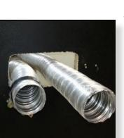
Cut flue exhaust tube (hot tube) to length (Approximately flush with wall exit). Connection plate will sit against wall.
