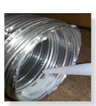
Apply an 8mm thick silicon bead fully around heater connection approx. 10mm from the top.
