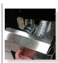
Assemble condensate drain and attach to pipe exiting wall. PVC pressure pipe cement must be used.
