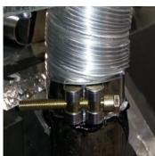
Slide flue onto connection spigot fully.
