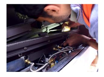
Undo gas connection pipe at end of burner. (15mm and 16mm spanner required)
