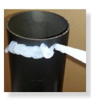
Recommended Silicon – Non-acetic, neutral cure 150degc or higher temperature rated. Bostik RTV 926 or similar.
