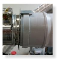
Ensure ends are burr free and round, test fit flue will fit over connection.
