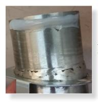
Apply sealant to flue inner and connector.
