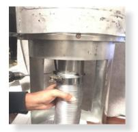
Slide flue onto connection spigot fully. Tighten clamp fully. Wipe excess silicon, visually check connection to ensure connection is fully sealed.
