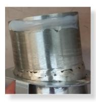
Apply sealant to flue inner and connector.
