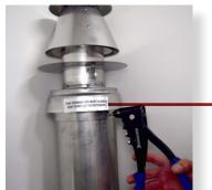
IMPORTANT- Apply silicon bead between inner connection of cowl and flue pipe to seal inner flue to cowl. Outer does not require sealing.
