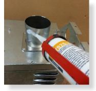
Apply an 8mm thick silicon bead fully around the lower fan connection spigot approx. 10mm from the end.
