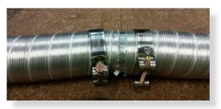
Slide each flue halfway onto connection joiner.
