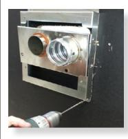
Locate wall mounting bracket into position and affix to wall.
