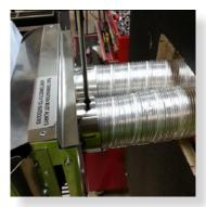
Feed air intake flue into connection, ensure inserted 50mm. Fit retaining screw from below. Insulation must start as close to the gas space heater as possible
