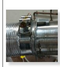
Fit flue clamp over flue (loosely).
