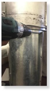
Flex collar and fit around the access panel. Socket the collar all the way up close to the air intake slots Ensure there is a rubber seal top and bottom of the collar.
