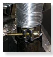
Slide flue onto connection spigot fully.
