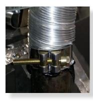
Slide flue onto connection spigot fully.
