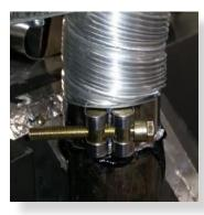
Slide flue onto connection spigot fully.
