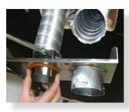
Slide flue onto connection spigot fully. Tighten clamp fully.
