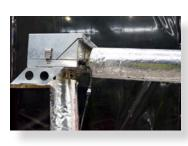
Insulation may be fitted prior and after the inline powerflue fan.
