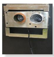
Feed power cable through bottom area of bracket.
