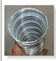
Check flue piece for correct shape and fitment onto appliance spigot.
