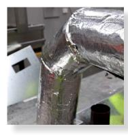
Insulation to be fully closed and sealed along length.
