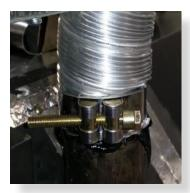
Slide flue onto connection spigot fully.
