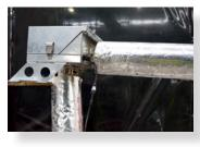
Insulation may be fitted prior and after the inline powerflue fan.
