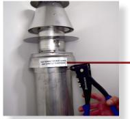
Screw or rivet in 3 places to hold in place.
