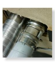
Push terminal into approximate position and affix onto wall
