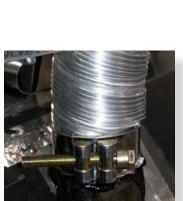
Slide flue onto connection spigot fully.
