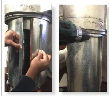
Flex collar and fit around the access panel. Socket the collar all the way up close to the air intake slots Ensure there is a rubber seal top and bottom of the collar.
