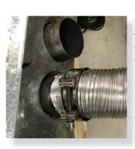
Slide flue onto connection spigot fully. Tighten clamp fully. Wipe excess silicon, visually check connection to ensure connection is fully sealed.
