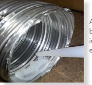
Apply an 8mm silicon bead fully around the inside of the flue end, both ends.
