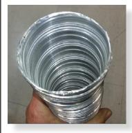
Fit air intake flue pipe to heater connection.
