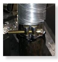
Repeat for air intake flue connection.
