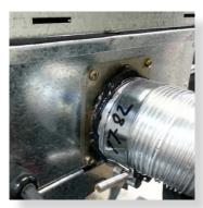
Slide flue onto connection spigot fully.
