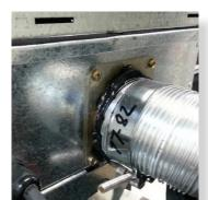
Slide flue onto connection spigot fully.
