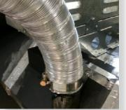
Clip flues as required to provide adequate support.
