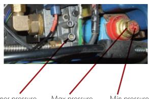
Burner pressure test point Max pressure adjustment nut
