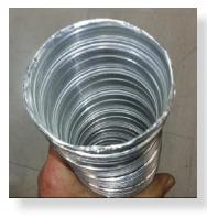
Ensure ends are burr free and round, test fit flue will slide over connection joiner.
