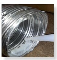
Flexi flue is in 7m lengths. A maximum of 2 lengths can be used.
