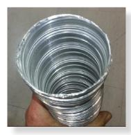
Fit air intake flue pipe to heater connection.
