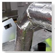
Insulation to be fully closed and sealed along length.
