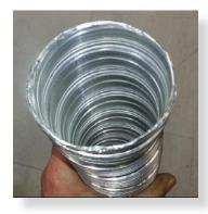
Cut flue to length to suit connection. Ensure ends are burr free and round, test fit flue will fit over connection.
