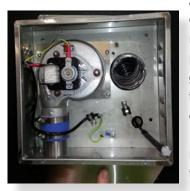
Assemble body main assembly onto wall mounting bracket, feed power cable through grommet hole prior to fitting. (refit 5 screws as shown and tighten) Main body assembly must sit flush up against the mounting bracket and seal.
