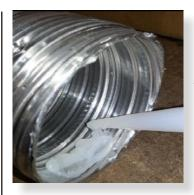
Apply sealant to flue inner and connector.
