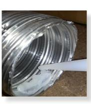
Apply an 8mm silicon bead fully around the inside of the flue end (heater connection end)
