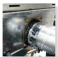
Slide flue onto connection spigot fully.
