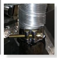
Slide flue onto connection spigot fully.
