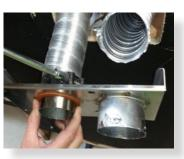
Cut flue exhaust tube (hot tube) to length (Approximately flush with wall exit). Connection plate will sit against wall.
