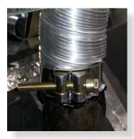
Slide flue onto connection spigot fully.
