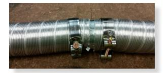
Slide each flue halfway onto connection joiner. Tighten clamp fully.
