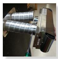
Feed hot exhaust flue into connection, ensure inserted 50mm. Fit retaining screw from below.
