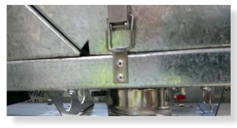
Repeat for connection to underside of fan module.
