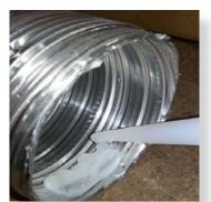
Apply an 8mm silicon bead fully around the inside of the flue end (heater connection end)
