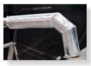
Bends were practical should be insulated, by cutting the insulation into segments and taping together. Failure to fit insulation on the exhaust flue may result in condensation failures with the appliance.
