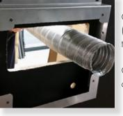
Cut air intake flue to length (Approximately 70mm through wall exit).
