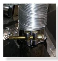
Slide flue onto connection spigot fully.
