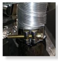
Slide flue onto connection spigot fully.
