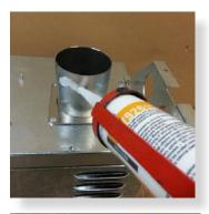
Apply an 8mm thick silicon bead fully around the lower fan connection spigot approx. 10mm from the end.
