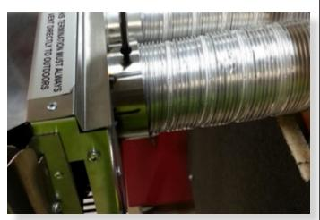
Cut inlet air tube. Flue must extend a minimum of 50mm past the exit face of wall.) It is recommended that the intake tube is cut slightly longer and pushed back into wall upon fixing of wall terminal. Allow flue movement between terminal and last intake flue hanging clip.
