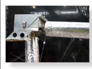
Insulation must be fitted prior and after the inline powerflue fan.
