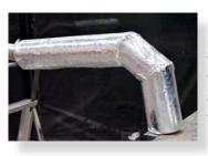
Bends where practical should be insulated, by cutting the insulation into segments and taping together.
