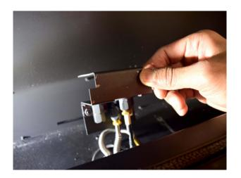
Remove pilot pipe fitting from pilot assembly.
