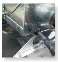
(Note 90° left connection is not available and must be done using the 90° right connection fan location and placing a bend in the flue to head in the LH direction. Fit 2nd flue clamp loosely onto the 65mm section of flue.
